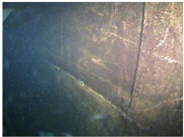
52) The sidewall has heavy mineral staining.
