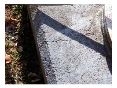
11) Minor crack in a leg foundation.
