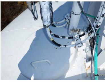
42) There is an antenna mounted 6 inches above the wet interior hatch.
