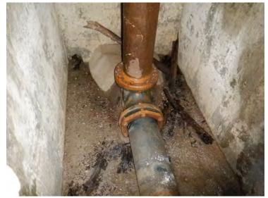
59) The coating on the pit piping is in poor condition.
