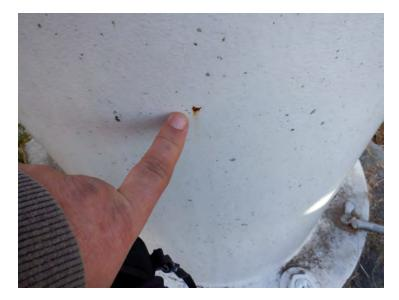
17) There are spot coating failures on the legs.
