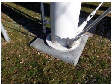
10) The exposed leg foundations are in good condition with minor deterioration.
